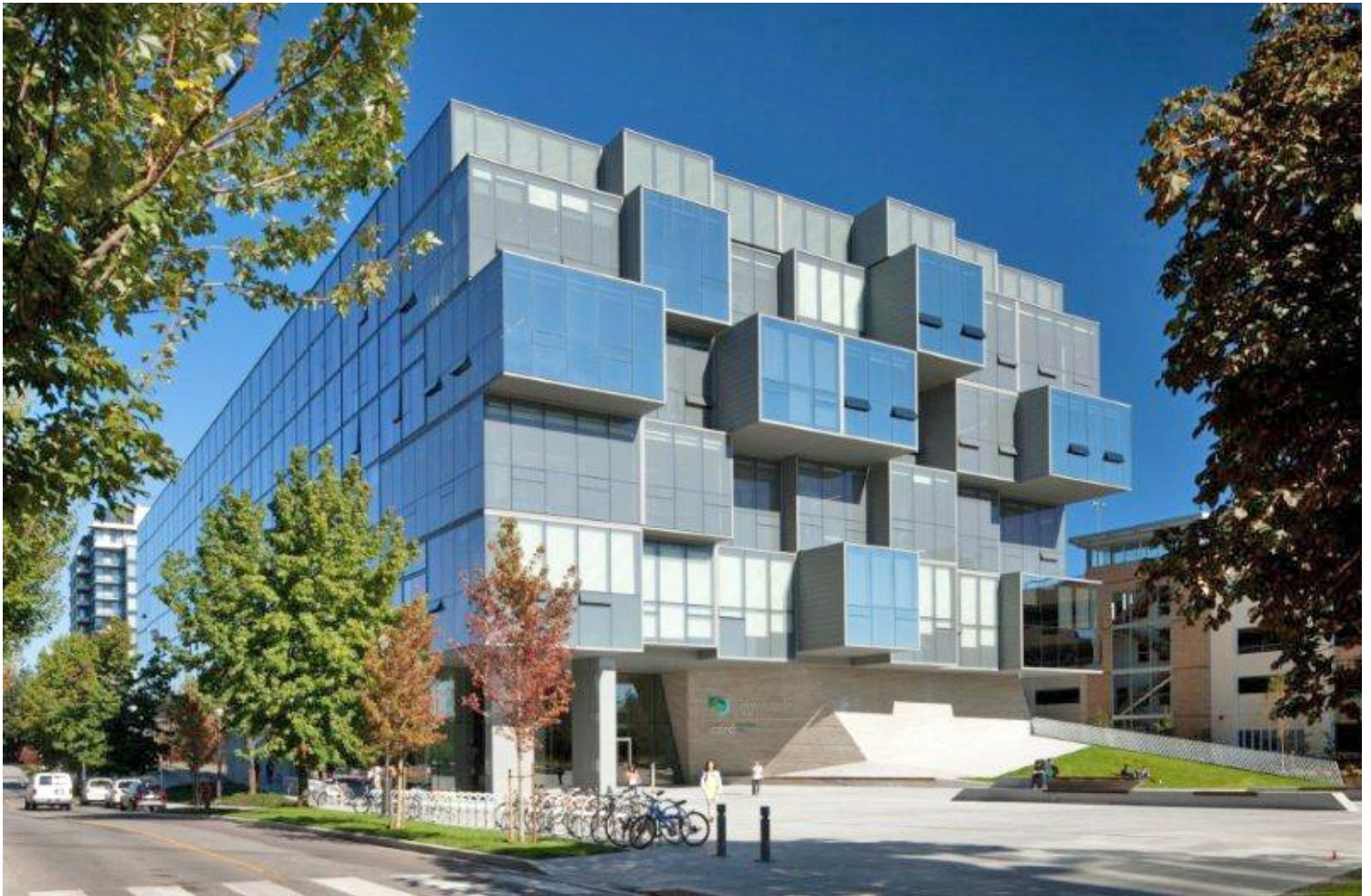
University of British Columbia - Pharmaceutical Sciences Building This 133 million dollar, 246,000 square foot state of the art complex, which will encompass all teaching, learning and research of the Faculty of Pharmacy.
